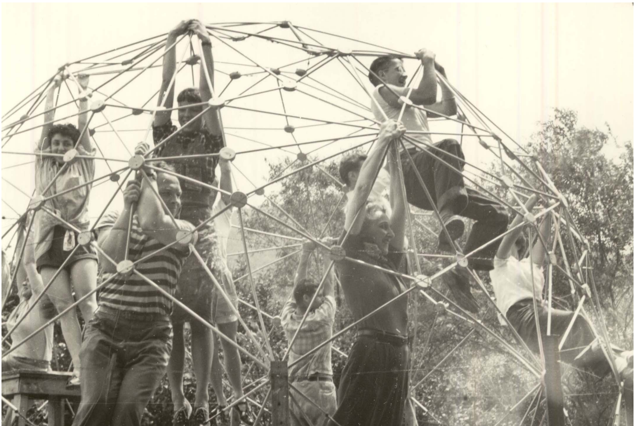
R. Buckminster Fuller, Geodesic domes (documentation of workshops), photo Masato Nakagawa, 1949, courtesy the Beaumont and Nancy Newhall Estate, Scheinbaum and Russek Ltd. and Western Regional Archives, State Archives of North Carolina
